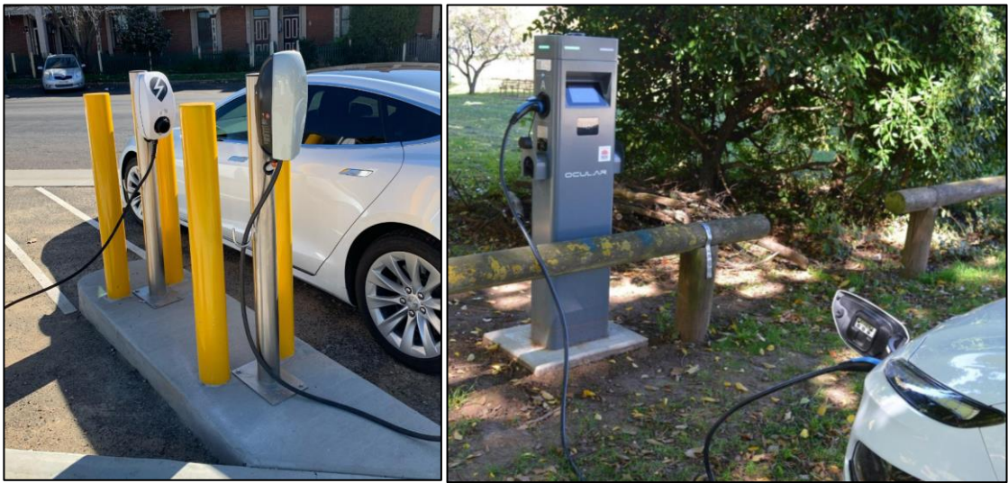
Bathurst Regional Council – Level 2 destination charging (‘wall mount’ left, dual port right)
